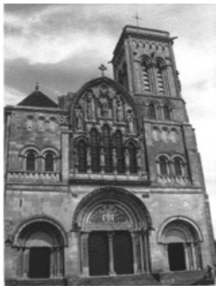
44. Vézelay, facade after restoration (photo author)
