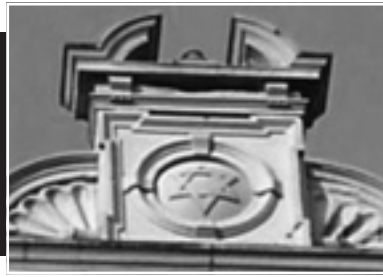
Fig. 2: Brewers’ star on a brewery in Mannheim, Germany. Photo: Michael Ohmsen and Google Earth
