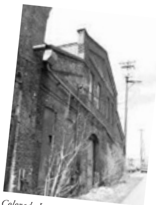
Colorado Iron Work today. Source: Photo taken by Brandy von Kaenel
