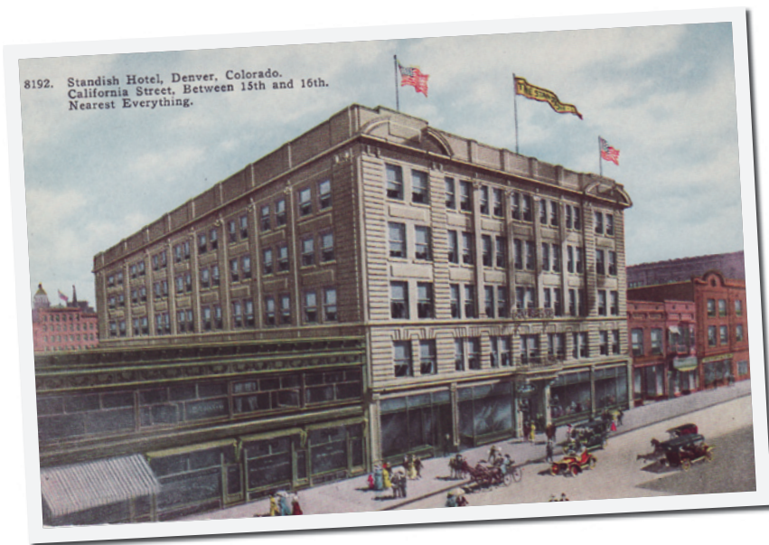
The Standish Hotel at 1530 California Street once housed stock show visitors such as the Sweeneys. It was demolished in 2008.
